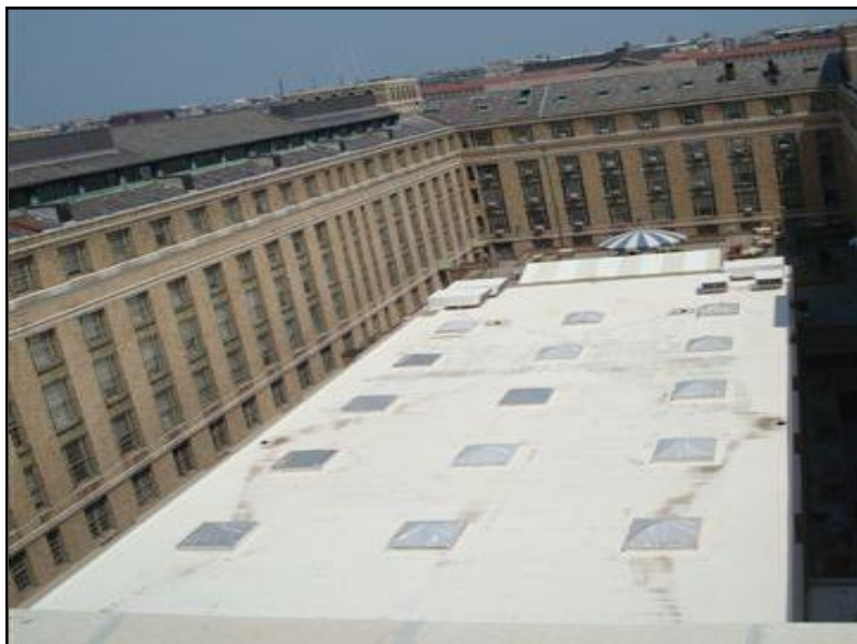
Court 2 in the South Building Waterproofing
